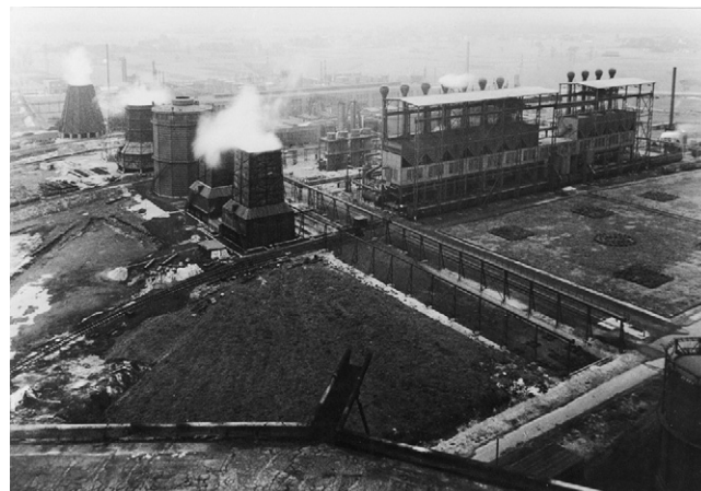
Fig. 1. Site overview Ruhrchemie FT production plant in Oberhausen, Germany, in 1930s: FT plant, cooling towers and a crane-way for catalyst filling. © OXEA Deutschland GmbH.
